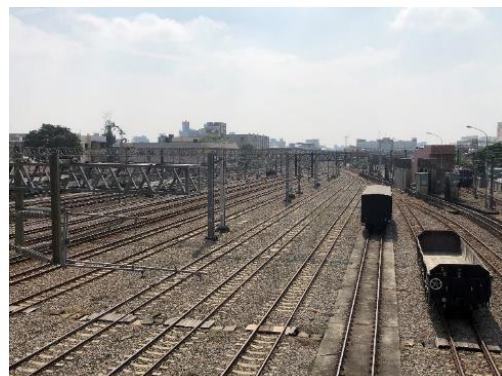
In the premises of the present Chiayi Station
