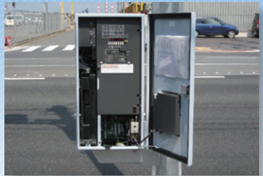
Local controller and emergency electricity supply unit
