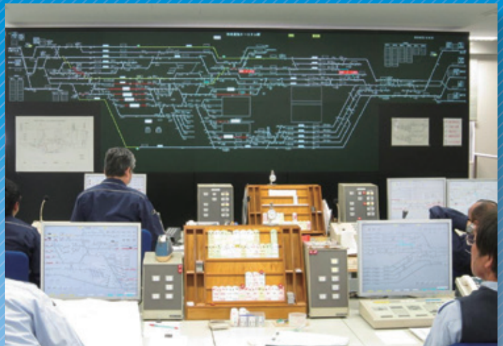
Relay interlocking equipment
