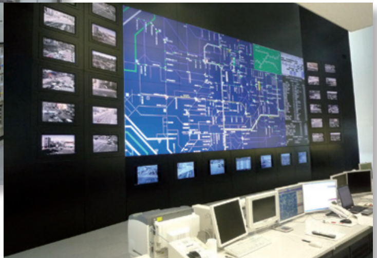
Traffic control center
