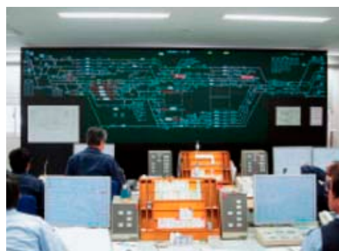
Relay control board and large-scale projector (Suita Freight Terminal Station)
