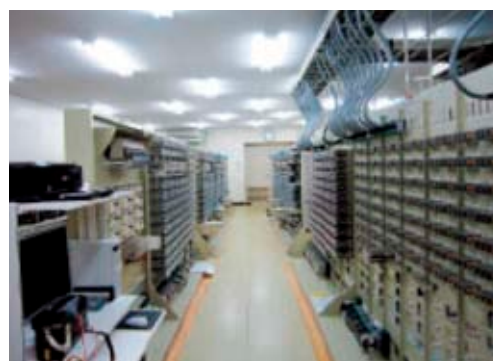
Equipment room (Kudara Freight Terminal Station)
